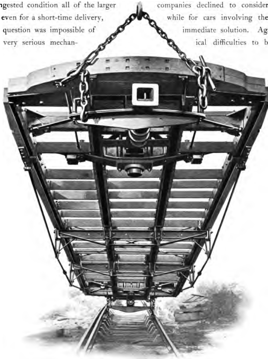
METAL UNDERFRAME OF PROTECTED WOODEN CAR
